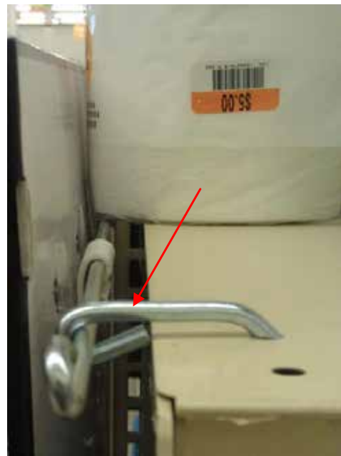
Power bar support hung on shelf structure.
